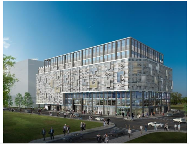
Cheongna Tetris parking tower new construction
